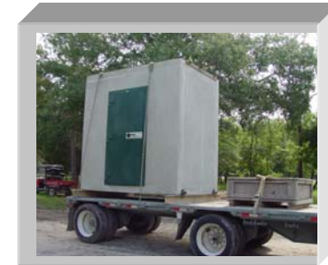
Delivery of concrete vault to residence.
