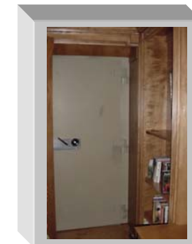
Vault entrance concealed inside a walk-in closet
