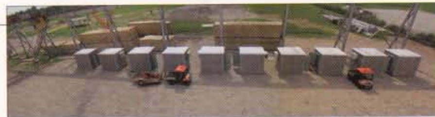
These Easi-Set precast concrete buildings, manufactured by Lonestar Prestress Mfg., Inc., were delivered in July as part of a City of Houston public works project. The buildings, engineered to withstand 140mph winds, house communications and Supervisory Control and Data Acquisition (SCADA) equipment for the Houston groundwater infrastructure upgrade project.
