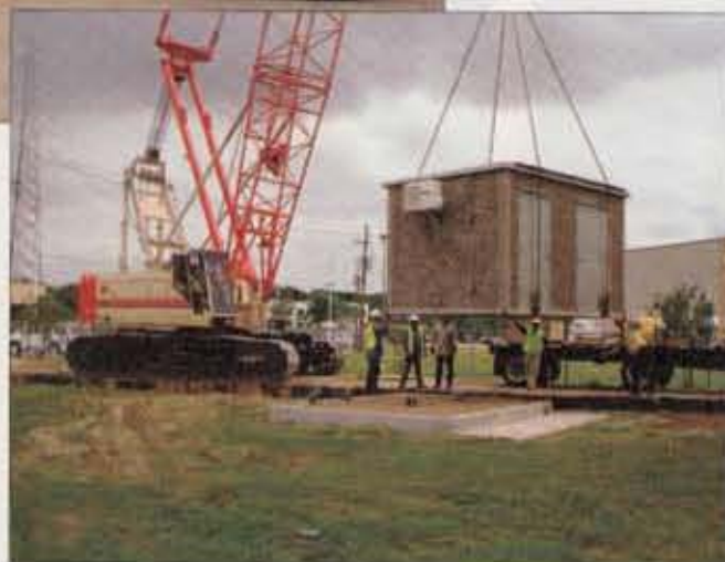
Lonestar Prestress' 10x14x8 foot Easi-Set building being offloaded at a Houston groundwater facility onto a prepared foundation consisting of precast retaining walls backfilled with pea gravel.
