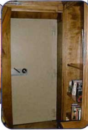
Fire rated tornado vault installed on house slab prior to construction.
